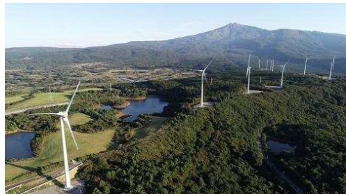
WE-02 Nikaho No.2 Wind Farm (Akita Prefecture 41.4MW 2.3MW×18 plants)
