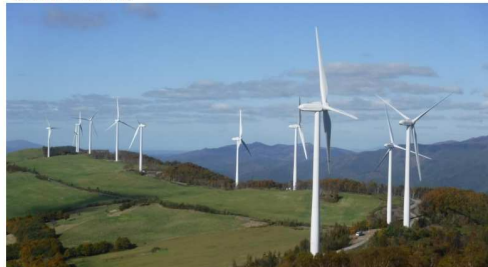
WE-03 Kuzumaki No.2 Wind Farm (Iwate Prefecture 44.6MW 2.0MW×16 plants & 2.1MW× 6 plants)
